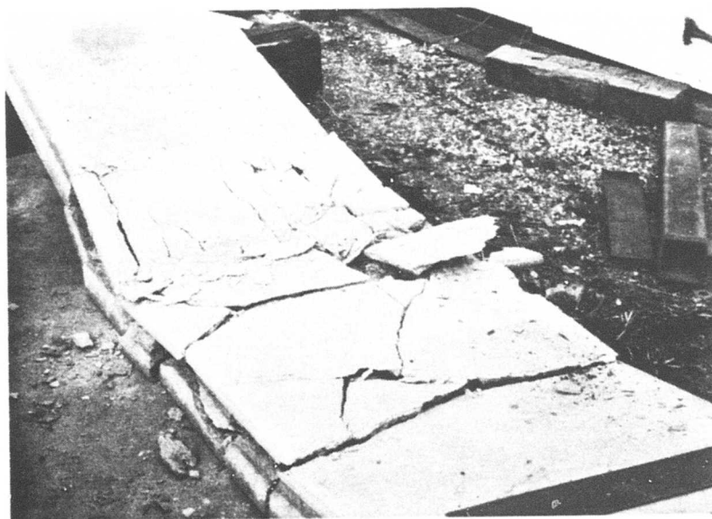
Fig. 2-10. Plank Failure After Load Was Removed.
