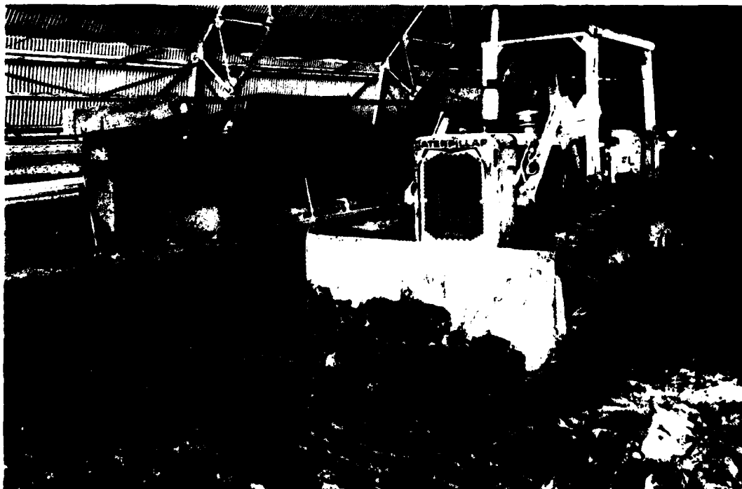
Photo 4. Bulldozer spreading heavy clay in test section
