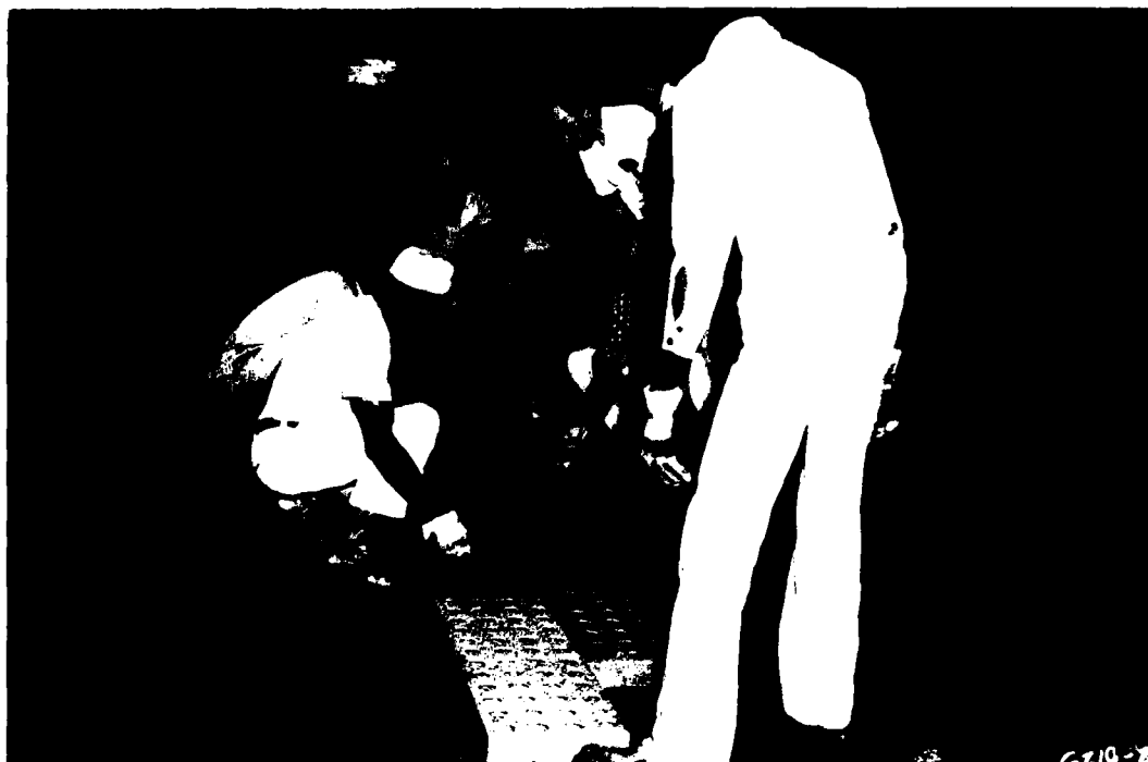
Photo 9. Two runs of Sod Saver Blocks being placed on test section, test I
