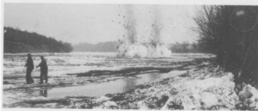
Blasting an ice jam
