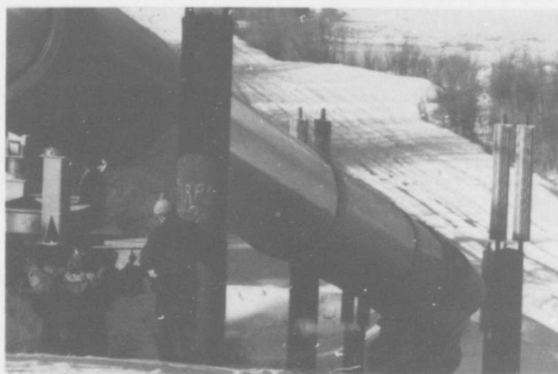
Measuring movement of trans-Alaska pipeline
