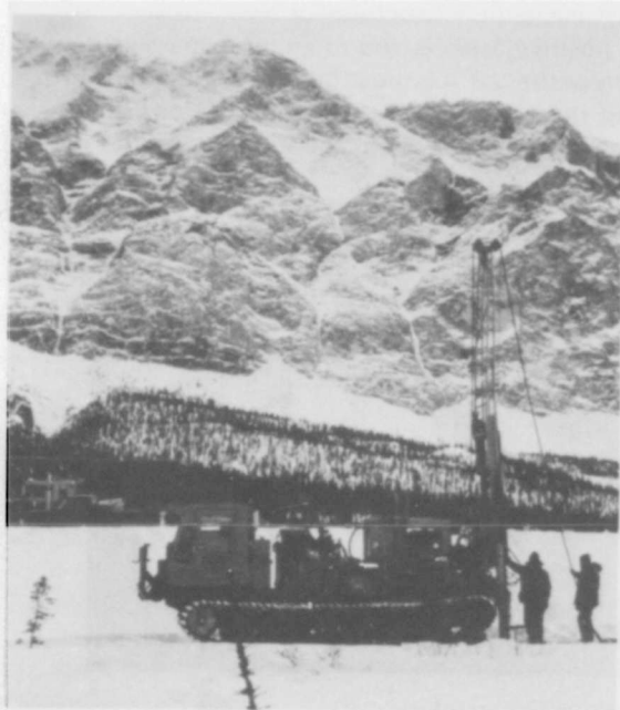
Installing a temperature-monitoring system in ground along trans-Alaska pipeline haul road
