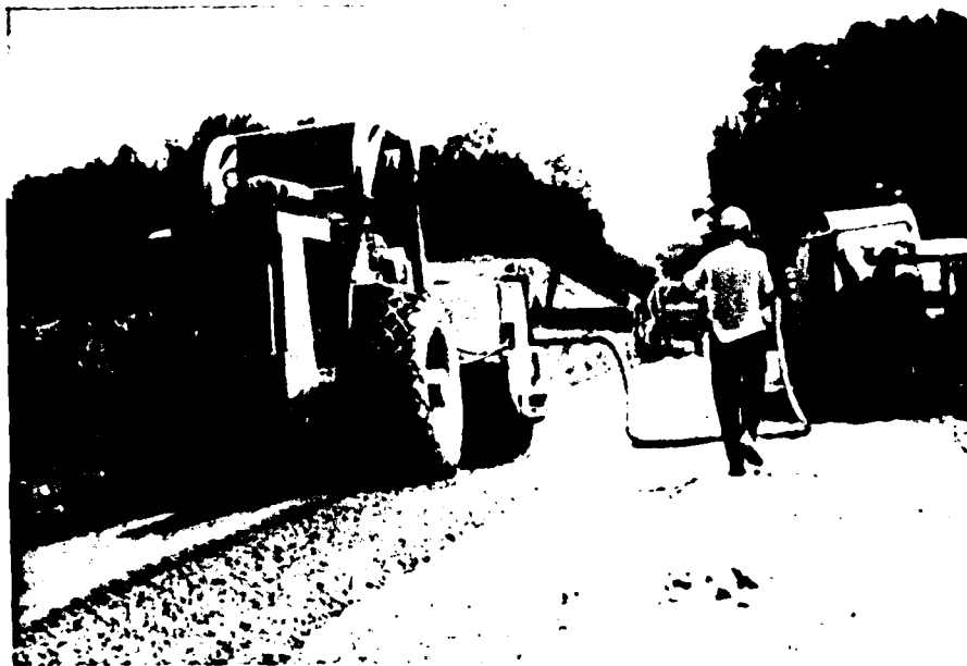
(13) Spray bar and water supply wagon used to add moisture to transition material. June 1975.
