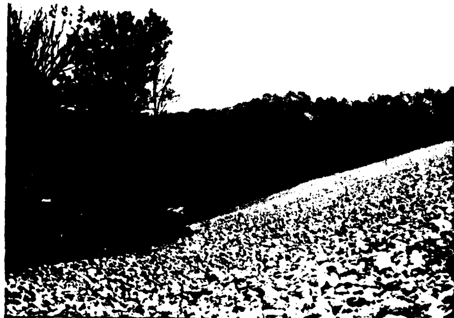
(25) View from right abutment to left abutment across upstream face of dam showing placed riprap. 4 Oct 1975.
