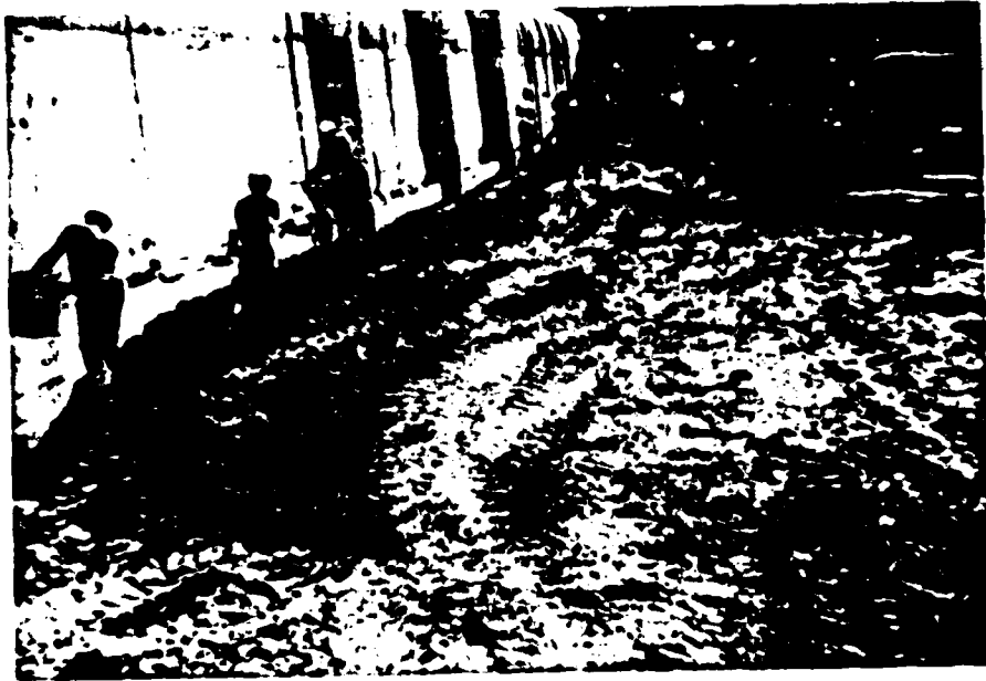
(7) Impervious embankment being placed along left side of conduit, and right abutment toe of dam 17 Sep 1974.
