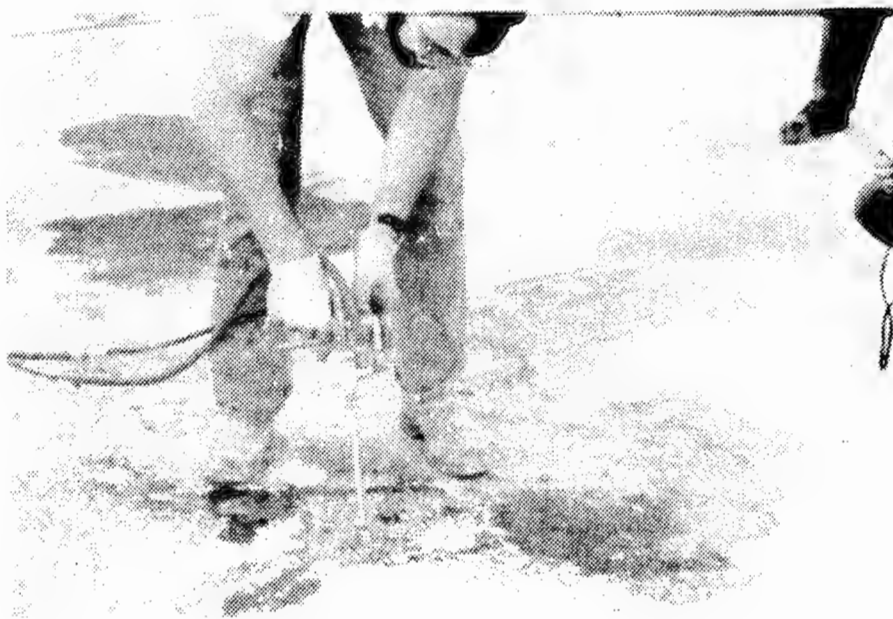
Figure 37. In-Line Mixing Gun.
