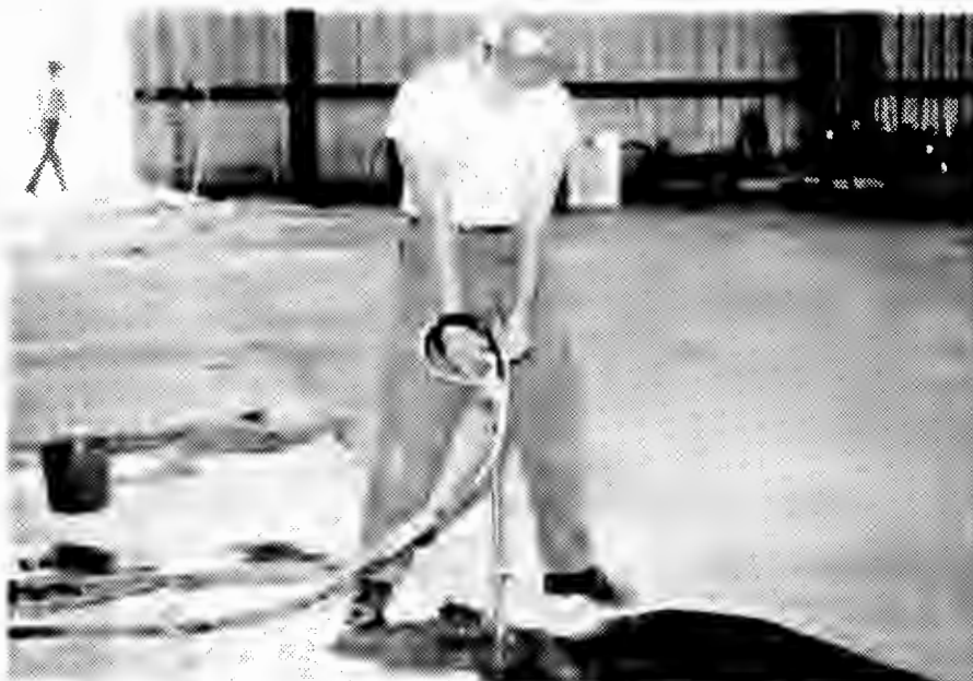
Figure 51. In-Line Mixing Gun Injecting Monomer Between Precast Slabs.
