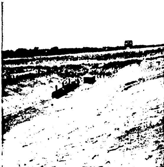
Photo No. 10 - View of discharge conduit and discharge channel during construction. Intake structure is in background. (June 1965)
