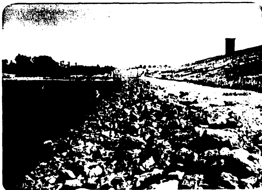
Photo No. 5 - Riprap with access berm on east embankment. Intake structure in background and water stage recorder housing at upper right. (Oct. 1979)
