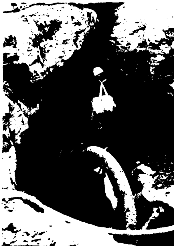
28. Solution channel Stillling Basin No. 6, Kv. Side of Pier 6. 27 Apr 78
