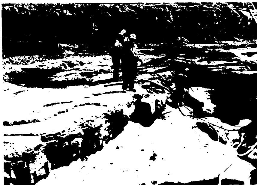
31. Stilling Basin No. 8, Showing rock "bridge" over solution channel after excavation, Looking downstream. 31 May 78
