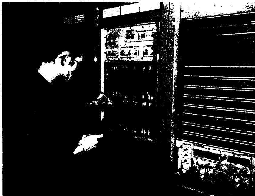
Plate 2. Student Removing Channel and Common Cards from the AN/GSC-24 Multiplexer Prior to Programming
