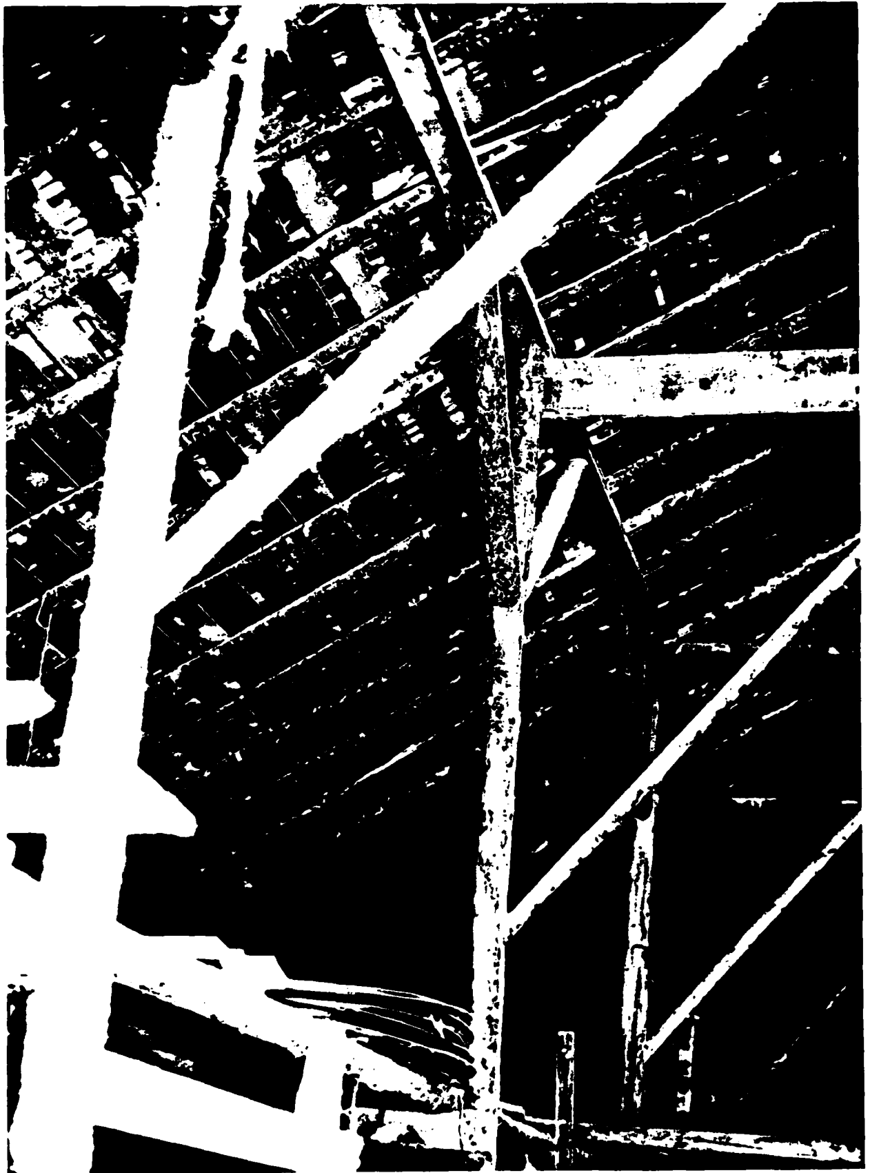
Fig. 3. Black Pine Timber Framing of Sheep Shed Owned by Terry Thompson
