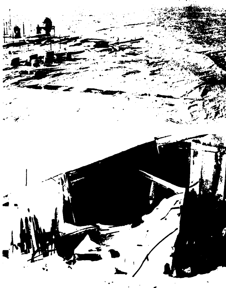
Figure 58. Bullen Point DEW Line Station, April 1979. Arrow points to garage damaged by ice and also indicates the direction of onshore ice movement.
