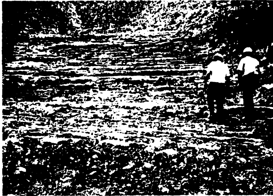
7. Typical right abutment cutoff trench foundation (5/27/72).
