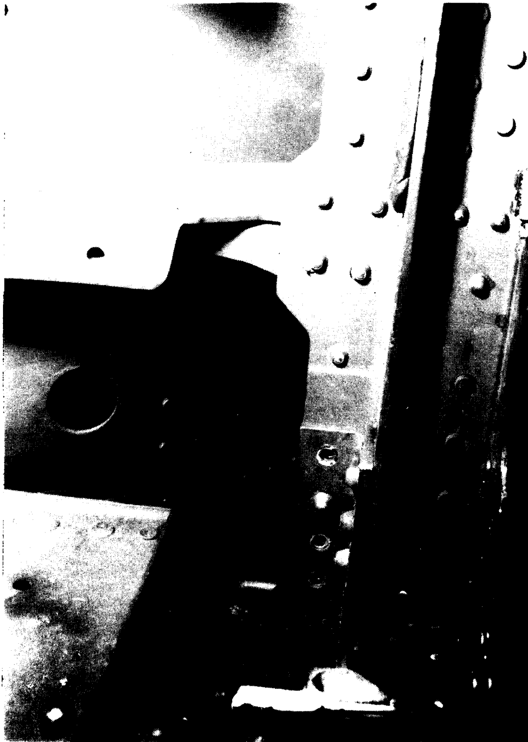
Figure 39. Rivets Missing from Splice Angle
