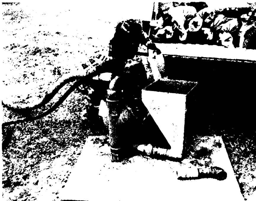
Figure 17. Pumping premixed, bagged slurry with Wilden M-8 diaphragm pump
