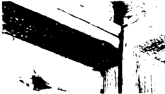
Figure 9.--Cold-weather condensation in corner of crawl space; the lumber had recently been installed to replace decayed lumber. The condensation, which continued and threatened further decay, was easily eliminated by laying an inexpensive vapor-resistant cover on the damp ground
