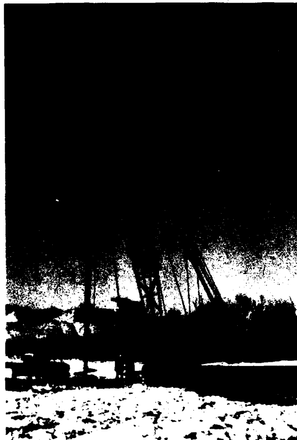
PHOTO NO. 4. Hole D-2 being drilled with a crane mounted drill. 12/4/73
