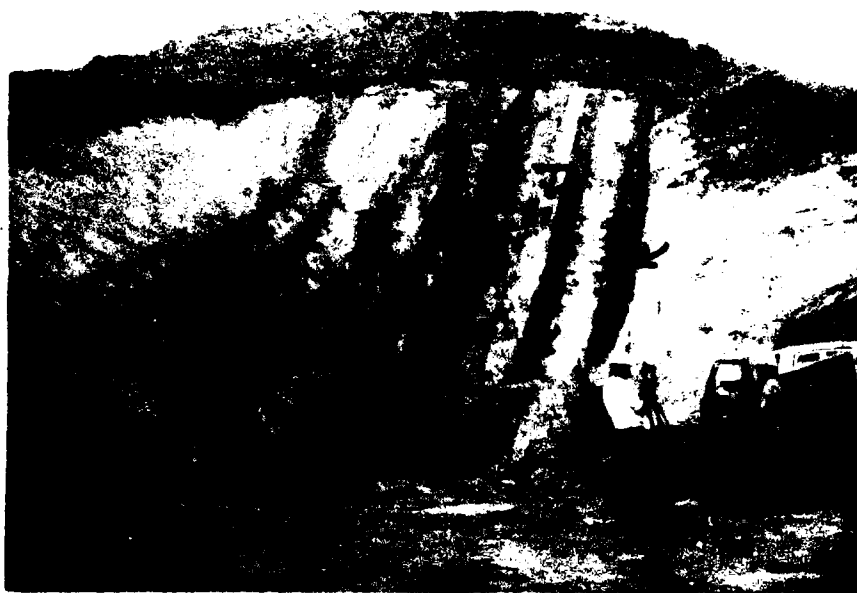
PHOTO NO. 75. Backslope of Mine #1 excavation, showing openings of drifts, raise, and a crosscut into coal seams. Looking south. 6/21/77.
