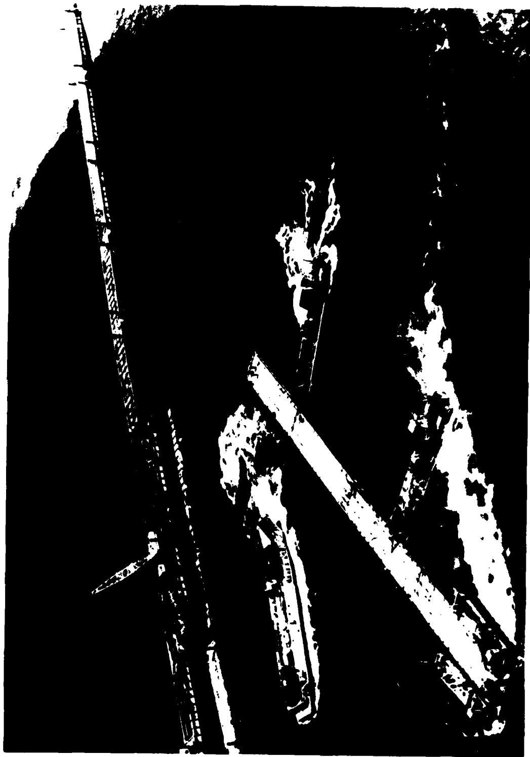
Figure 21 - ELCAS Extending from the Beach to Beyond the Surf Zone
