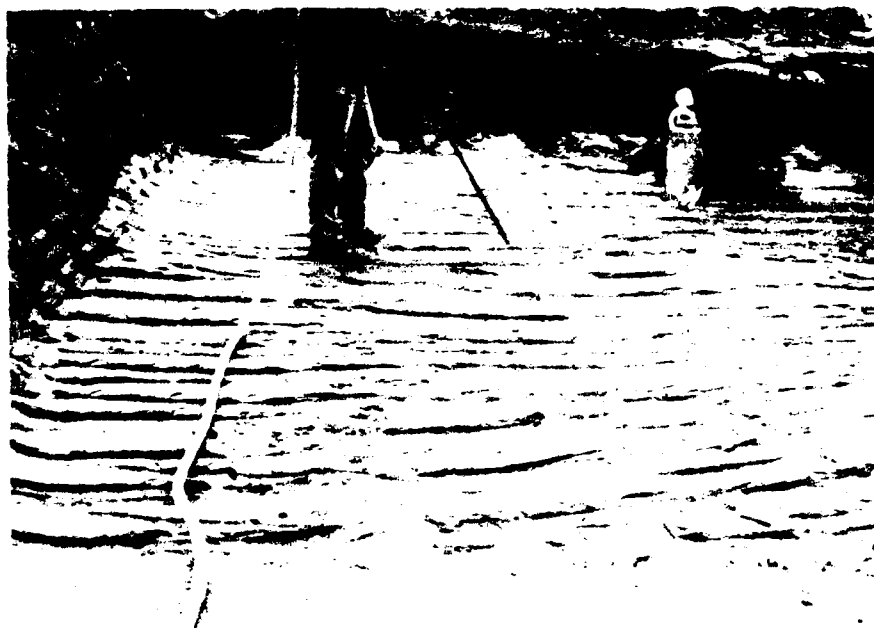
Fig 58 Stilling basin foundation. Station 28+78 31 Jan 81
