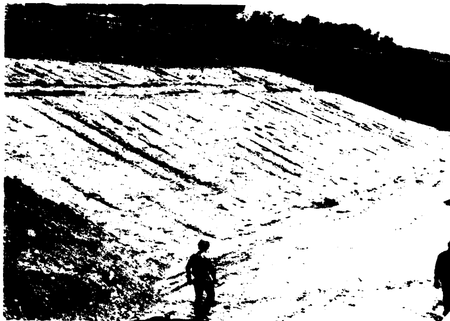
Fig 82 Excavation slope right of conduit. Station 24+00 - 25+20 26 Aug 81
