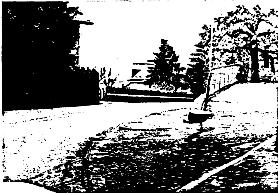
Figure 37: This intersecting road from the right side, located just behind a curve to the right, is improper because a maximal preview time of only 1.5 s is allowed. This time is insufficient for an adequate reaction to any unexpected event perceived at the last moment.
