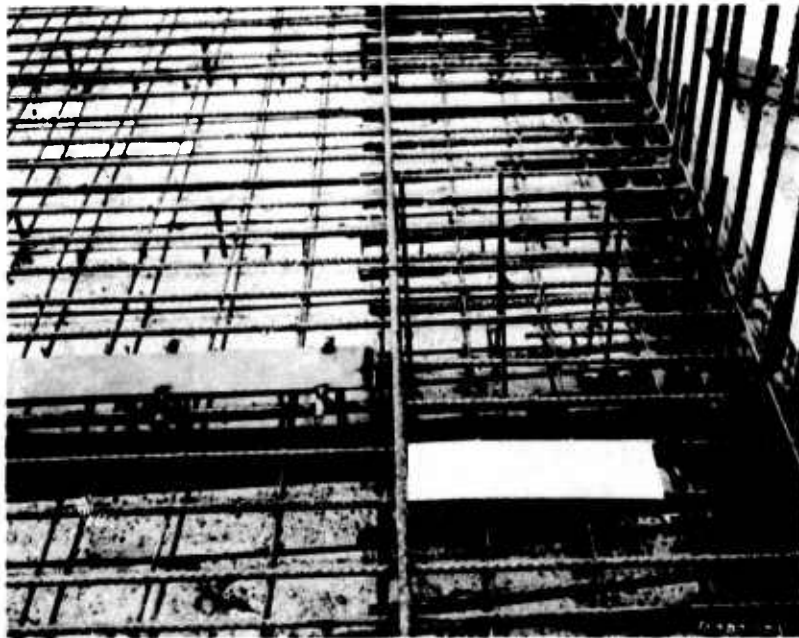
b. Detail at blast door bulkhead.
