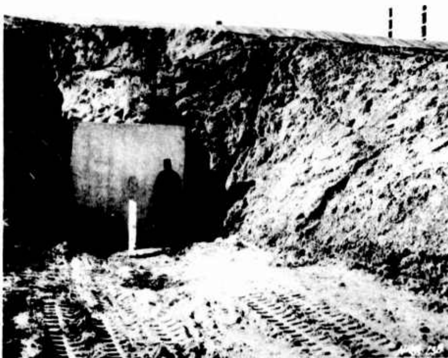
Figure 2.31. Concrete slab placed in donor bay entrance.
