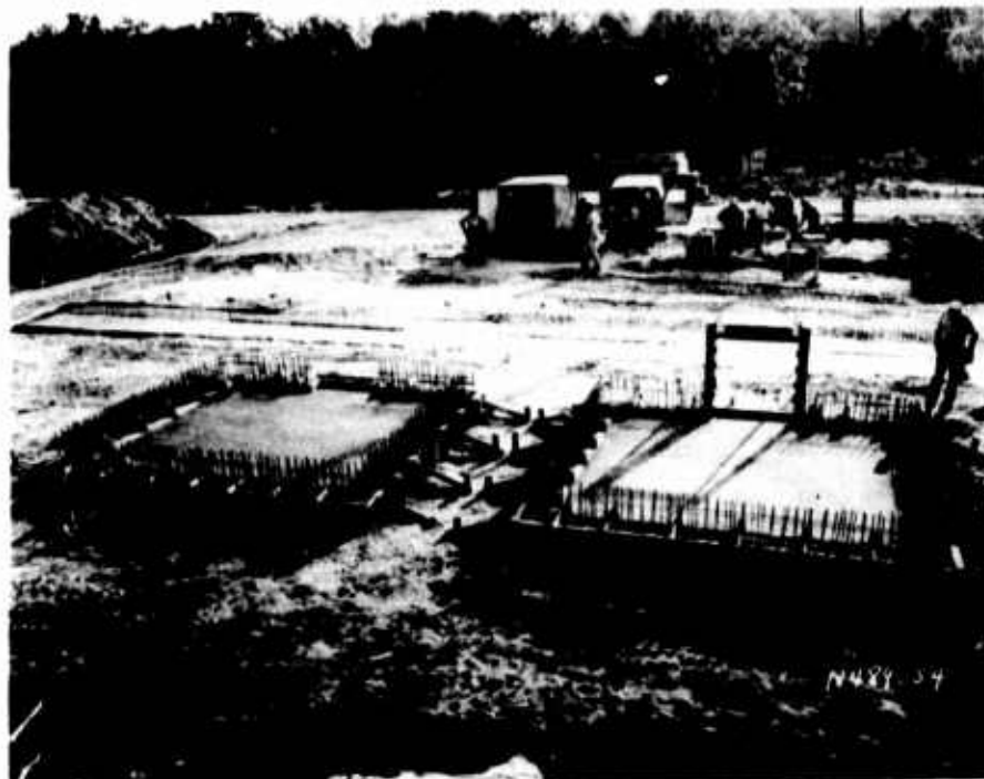
Figure 3.12. Completed bay floors and retaining wall footing.
