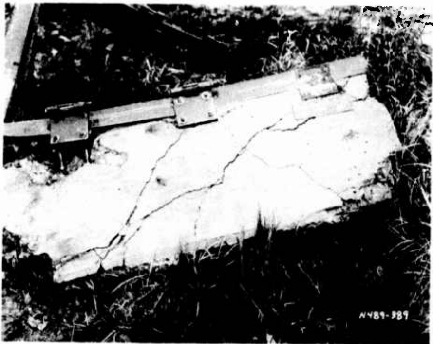
b. Detail of north side.
