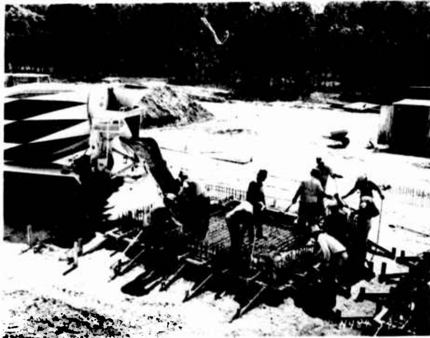
Figure 3.11. Concrete placement in bay floor.
