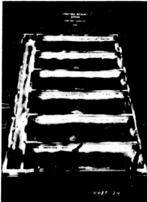
Figure 3.27. Internal construction of inactive blast door leaf.
