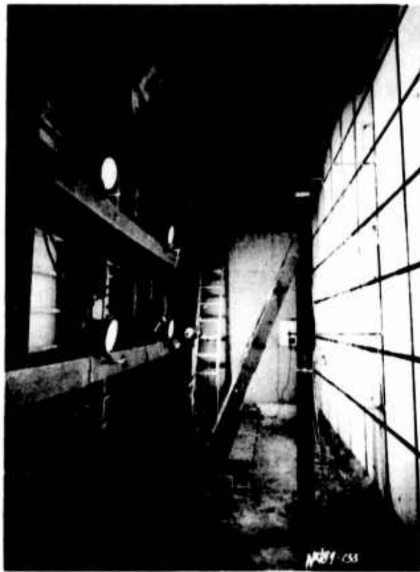
Figure 2.29. Interior of acceptor bay.
