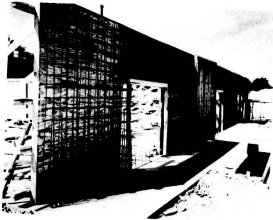
a. Overall view.
