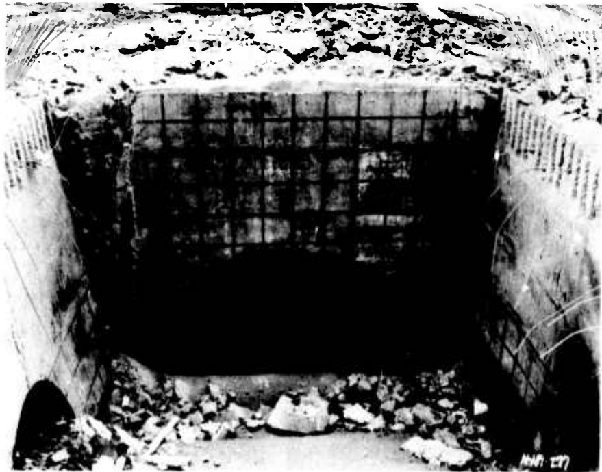
a. Overall view.
