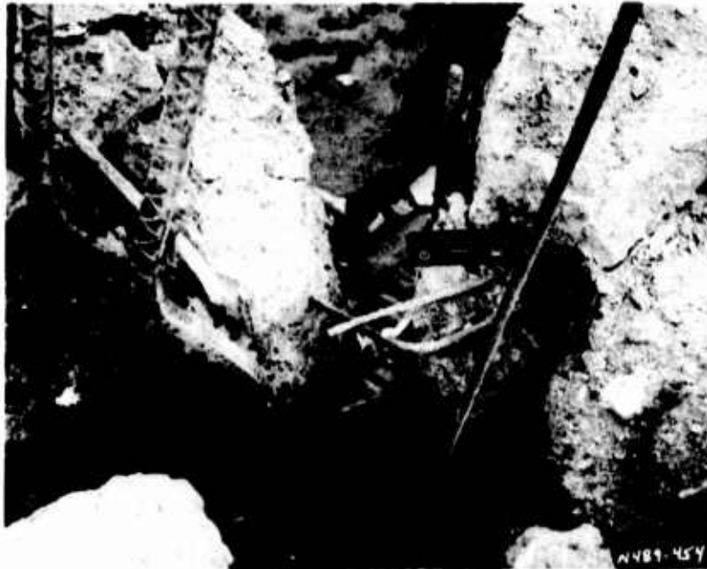
f. Exterior view of southwest corner.
