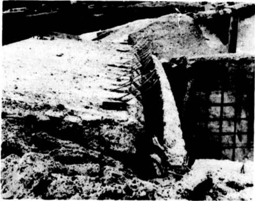
c. Detail of west half of roof slab.
