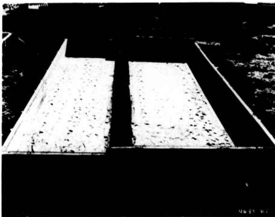
b. Acceptor bay formwork.
