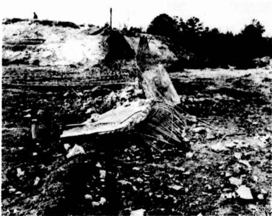
b. View facing west.
