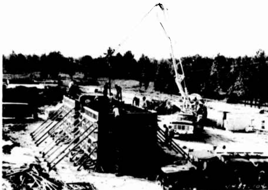
Figure 3.15. Concrete placement in bay walls.
