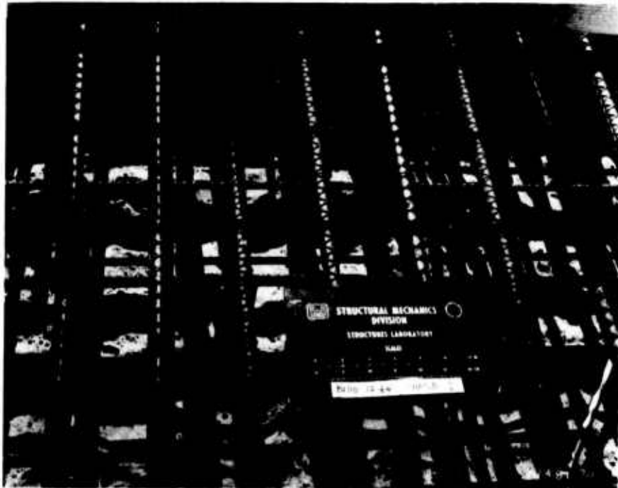
Figure 2.10. Detail of slab reinforcement.
