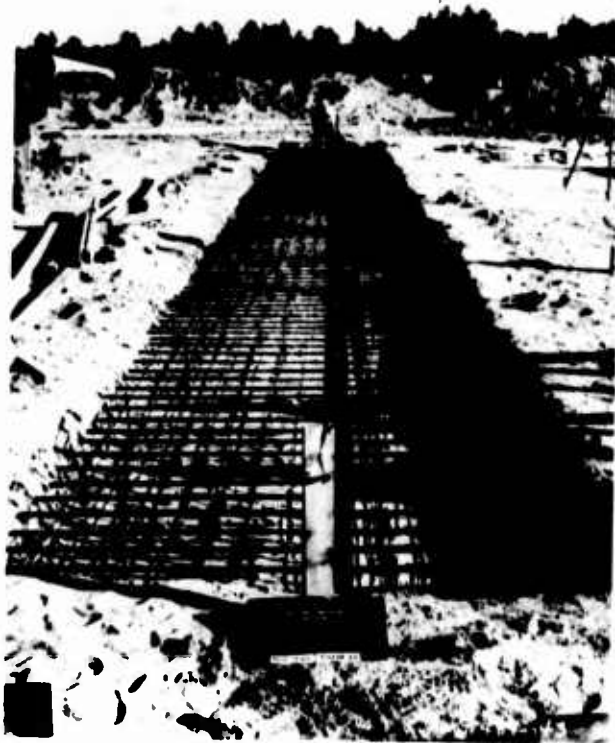
a. Overall view.
