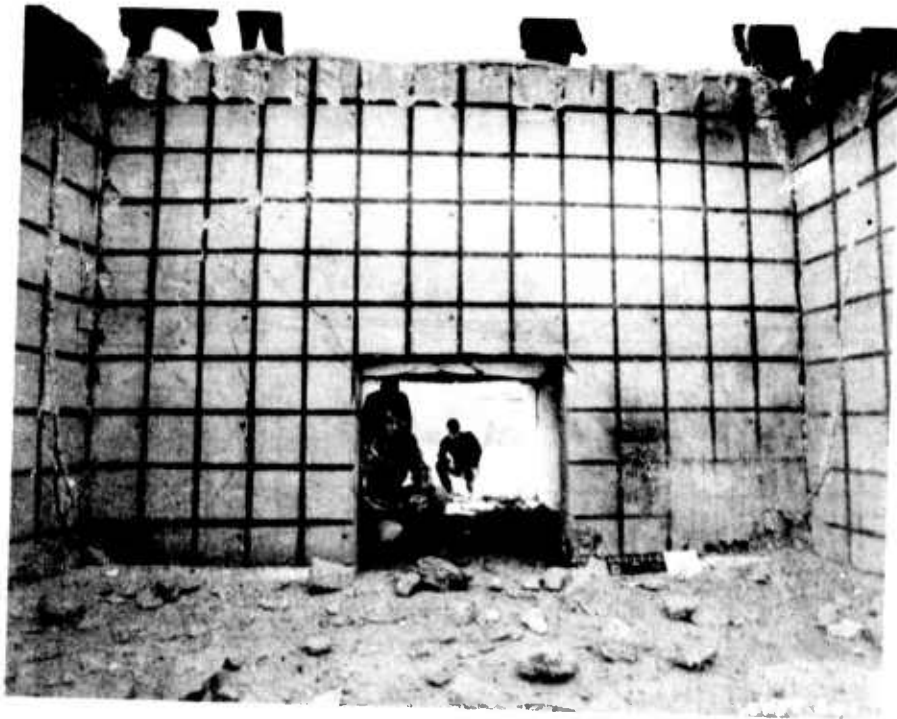
a. Overall view.
