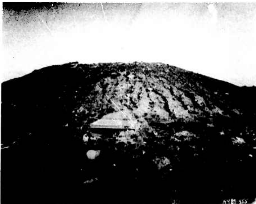
Figure 4.10. West slope with W grid.
