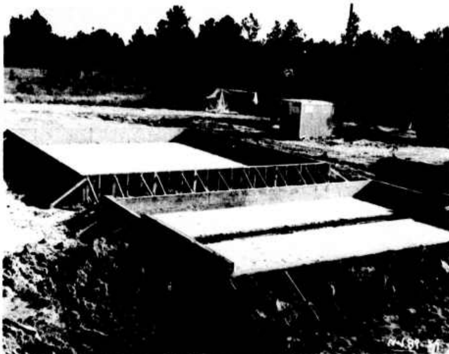
a. Donor and acceptor bay formwork.
