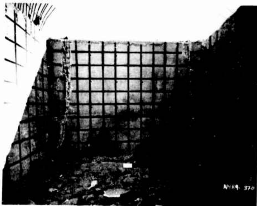
a. Overall view.
