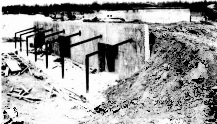
b. Native soil placed around bays.
