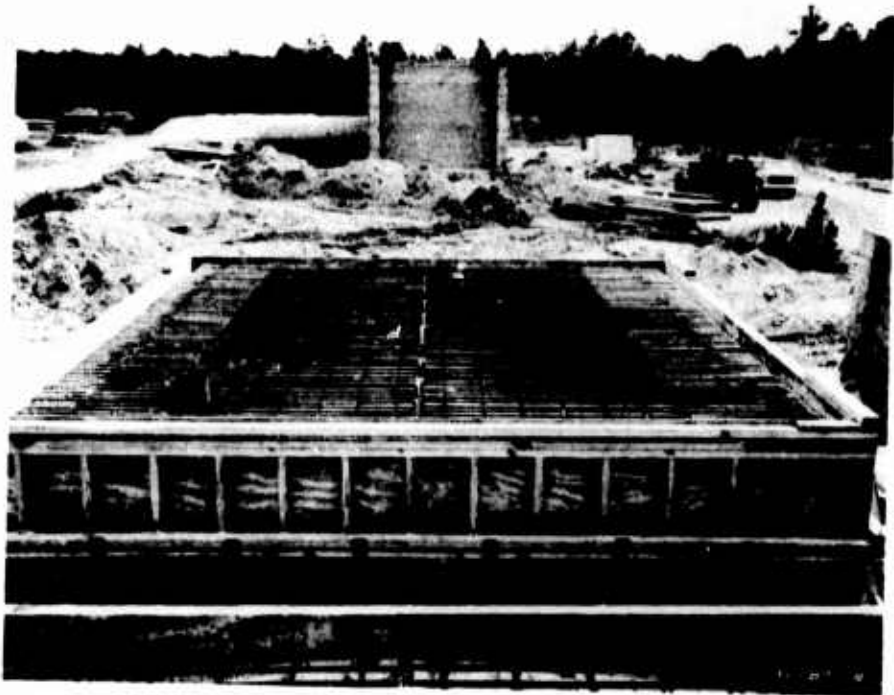
a. Overall view.
