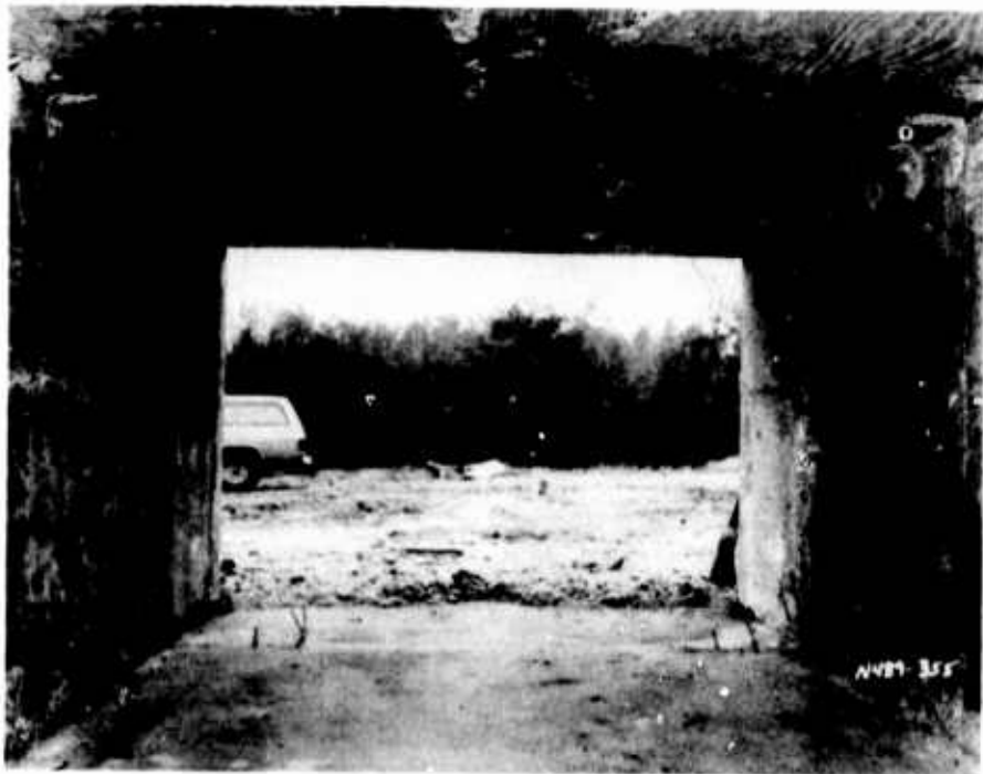
b. Internal view at door bulkhead.
