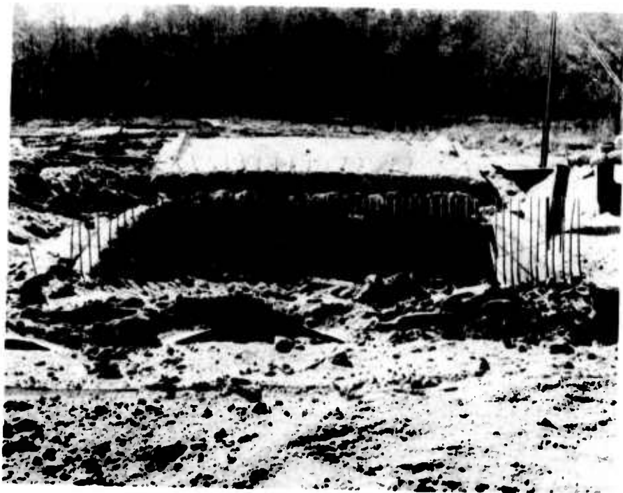
b. View facing west.
