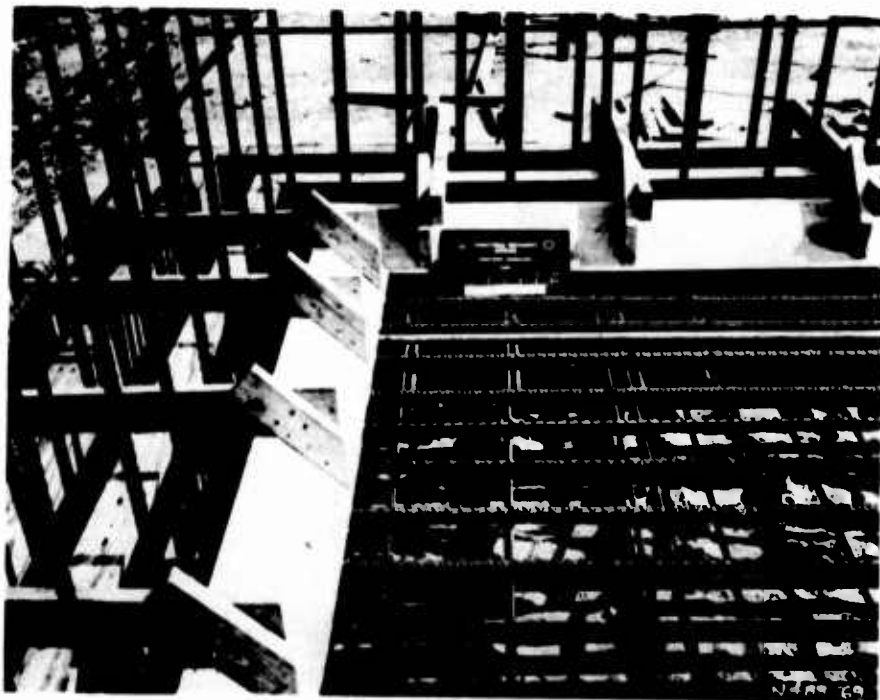
Figure 2.9 Corner detail of donor slab reinforcement.
