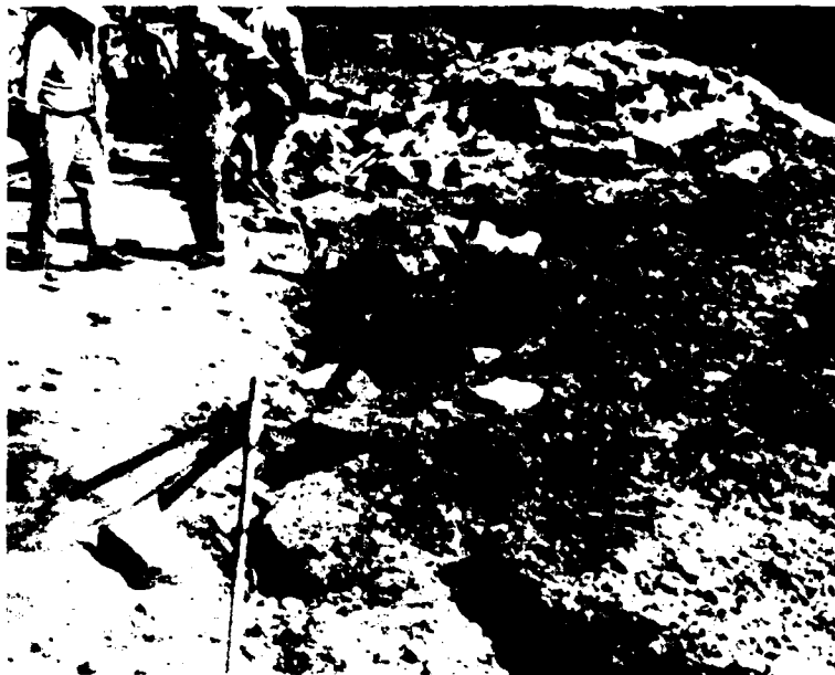
3. Milford Dam, October 1962, Neg. No. 294-P4-5. Test shot results for pre-split blasting.
