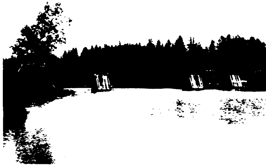
Figure 21. Ice-holding timber cribs in the Narragaugus River, Maine.
