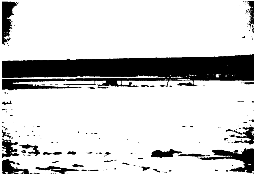
Figure 20. Rock-filled scow stabilizing the ice cover in Soo Harbor, Michigan.
