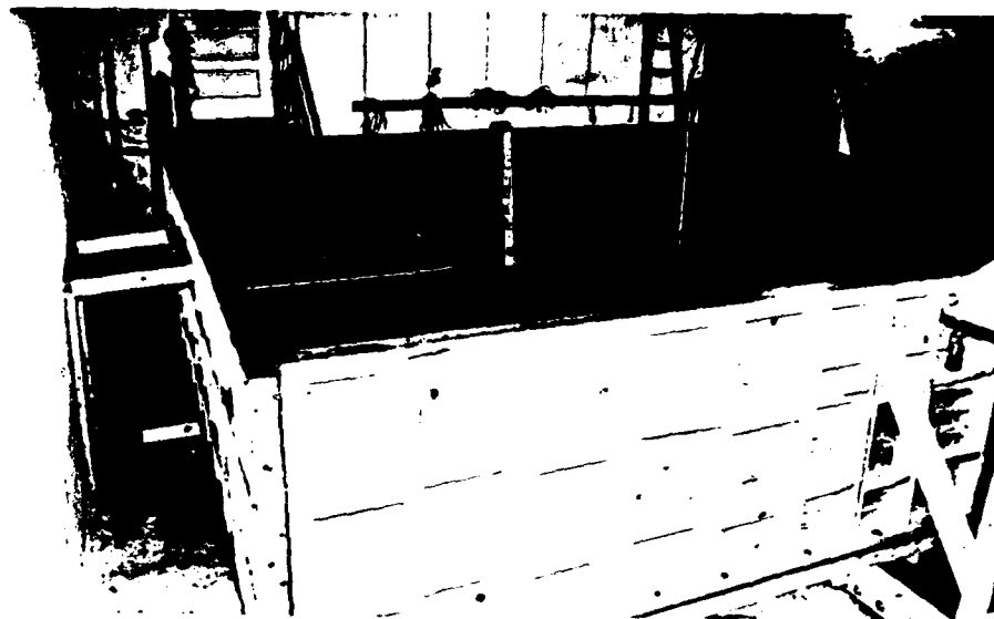
FIGURE 2-2 Large Water Tank
