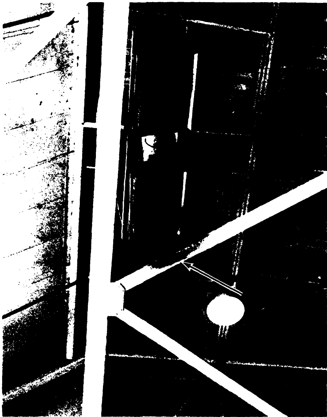
Figure 3. Damage to structural member caused by incorrectly mounted IR radiant heater.
