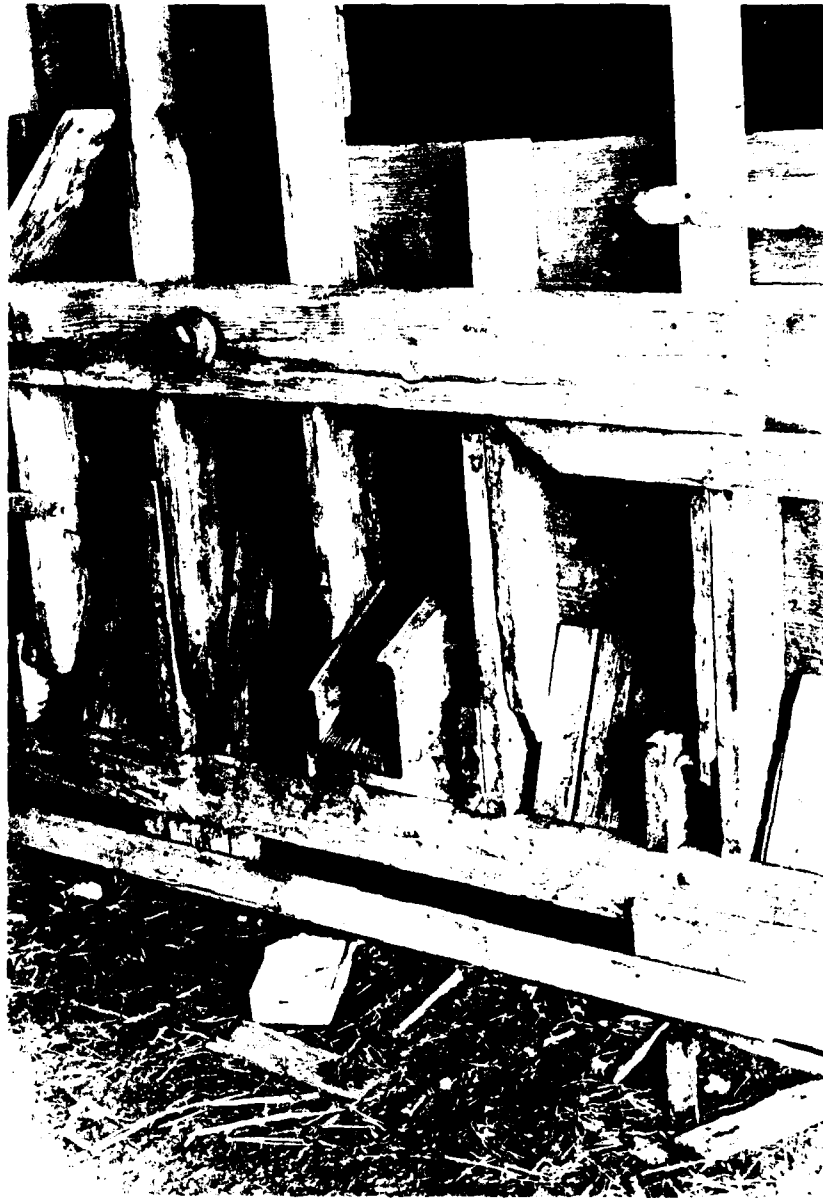
Figure 11-38. Architectural detail of the Holveck barn (exterior). Note chute for removal of grains, bolted end of stress rod which passes through crib.
