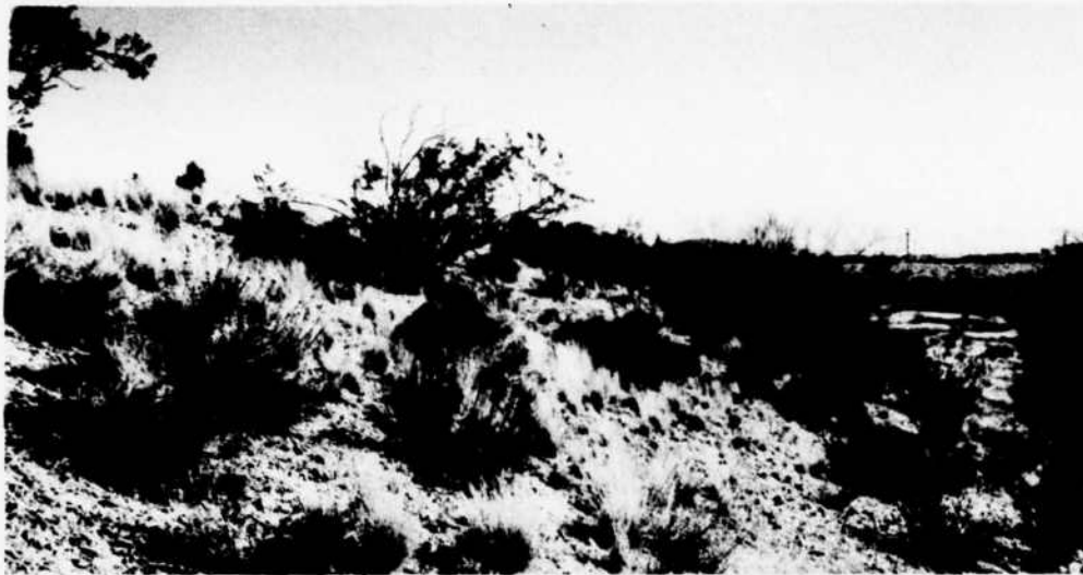
Photo 5. Grasses and Shrubs on Levee Walls Where Moisture is Scarce.
