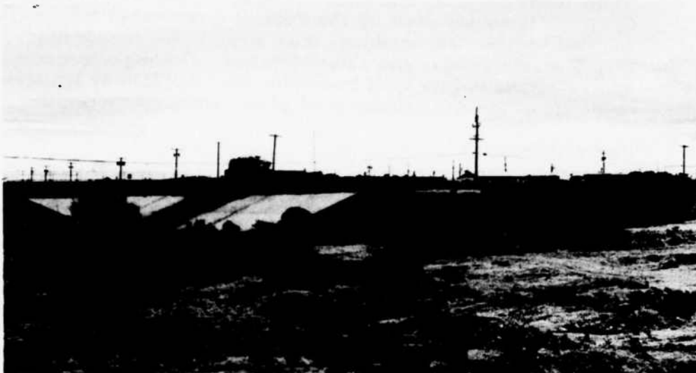
Photo 1. Looking East Toward the Inlet Channel of the Tucson Detention Basin.
