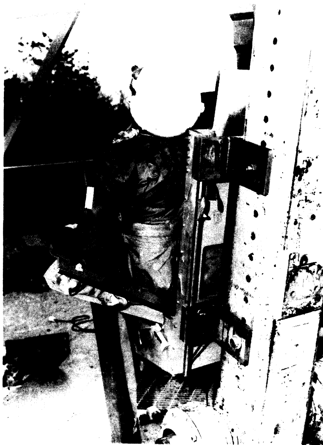
Figure 27. HELPS Attachment Failure
