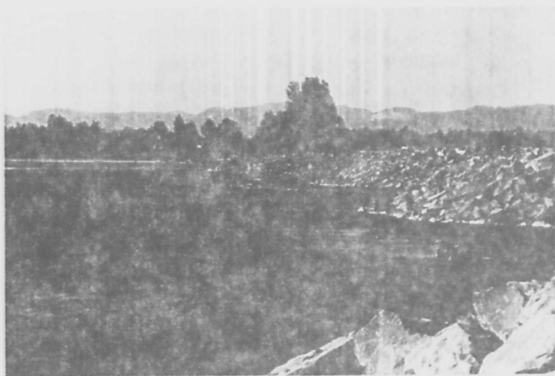
A. Looking Downstream From Dike 5
