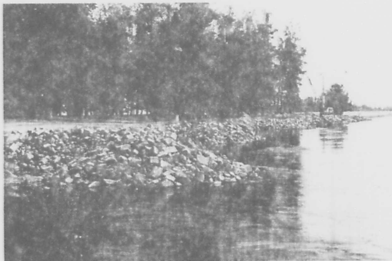
B. Looking Upstream From Dike 6
