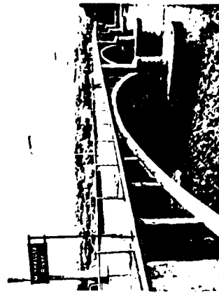
During high water, ice and debris caught behind the Mankato Bridge from up the Minnesota River and cause further flooding.
