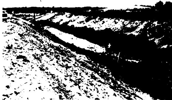
Figure 5. Cutoff trench, 1st contract: Backfilling (near) and sealing off water with fill (distant) along trench toes. Casing of large diameter auger boring in distance.
