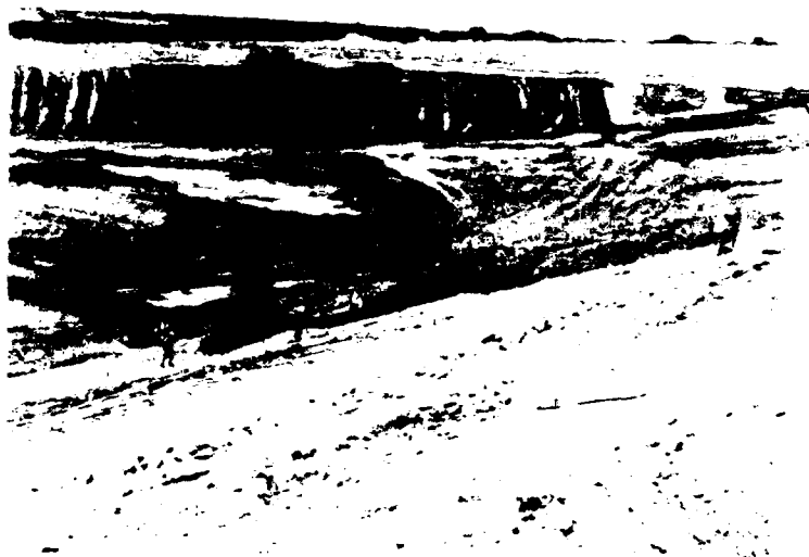
Figure 70. Spillway, 3d contract: View diagonally across spillway chute (downstream and toward the right sideslope). View shows granular refill (near), the chute work slab with anchors, and the drainage blanket and fresh excavation in the distance.
