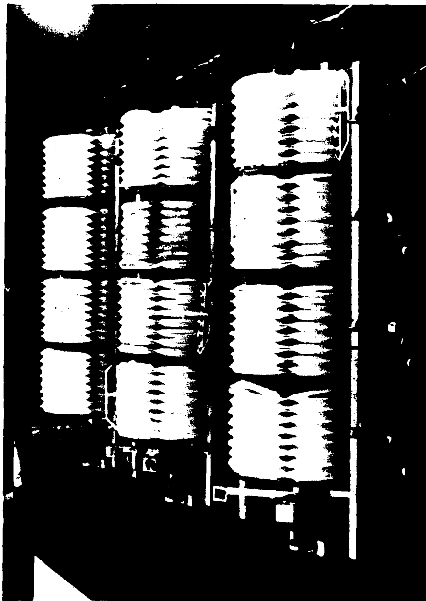
Figure 7. RBC treatment units before wastewater was applied. Flow was directed from top to bottom with the RBC in the foreground being the third stage for each wastewater to be processed.
