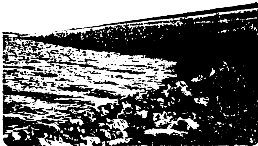
PHOTO NO. 11 - View of riprap slope protection on right abutment shoreline area. September 1982
