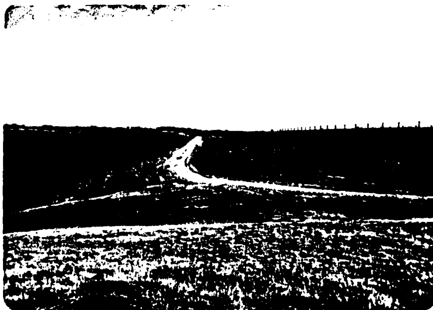
PHOTO NO. 6 - View of upstream embankment slope, crushed rock surfaced service road, and upstream slope riprap protection from the right abutment. September 1982
