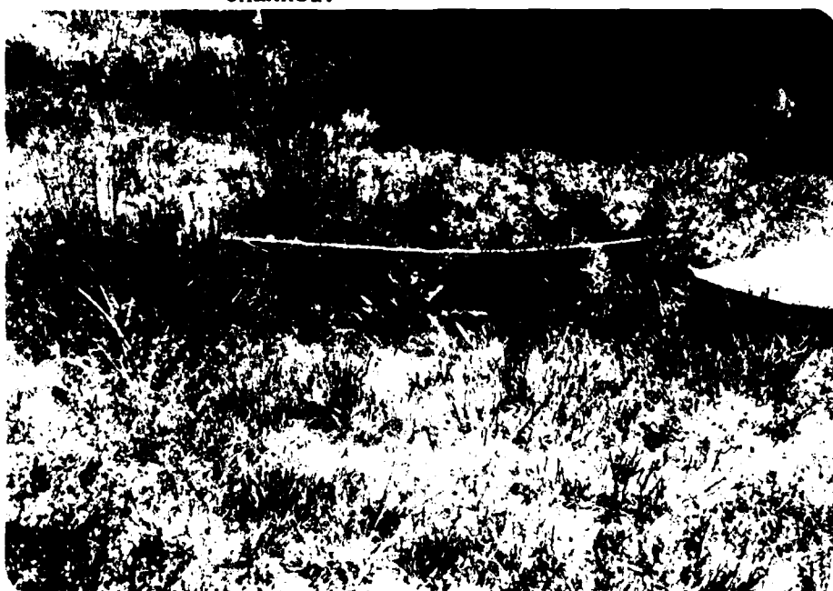
PHOTO NO.4 - Subsidence of ground surface in area over arch culvert. Note six (6) foot rule and unfolded plan.
