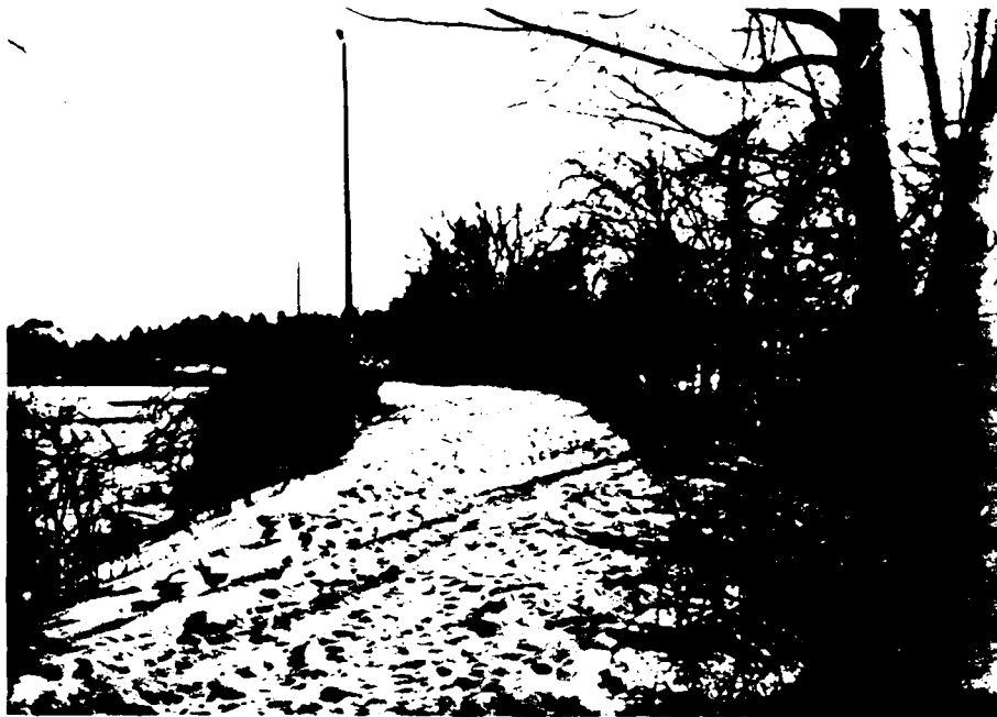
Photo 2 - View looking south along crest of dam.
