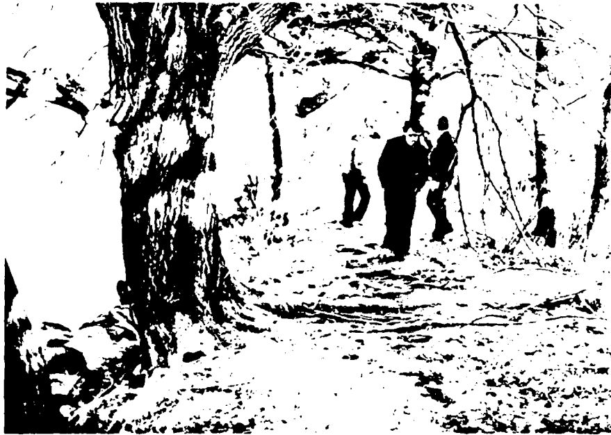
10. View along crest of dike
