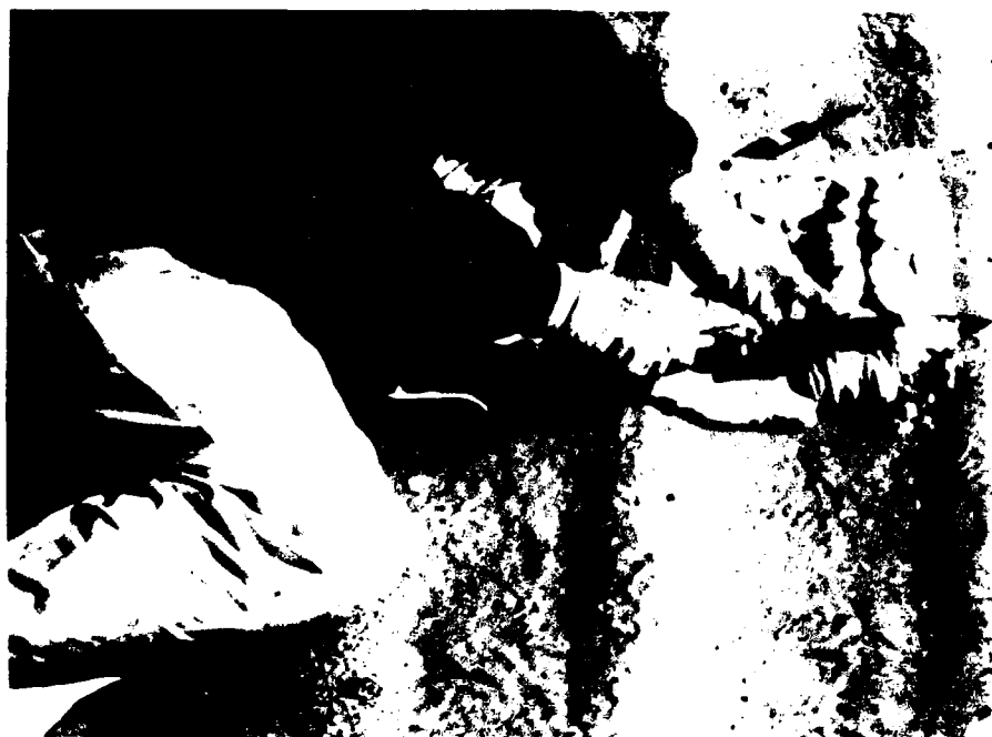
(d) New foam patch is shaped with a knife.
