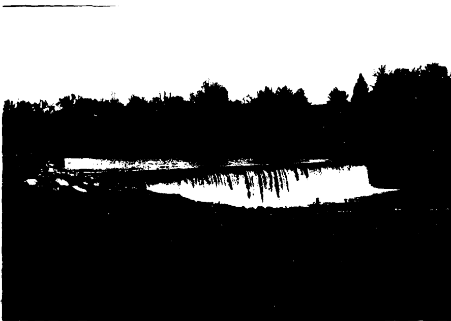
C-2 Spillway from right side of channel.
