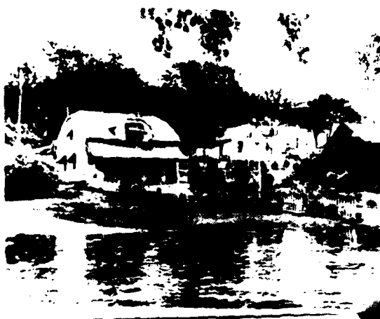
at 1209 West Conant Street September 1938
