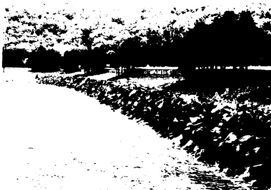
PHOTO 5 UPSTREAM FACE OF DAM
