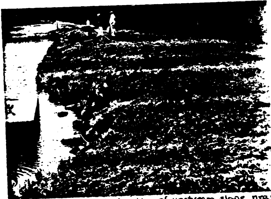
Photo 7 - Erosion and sloughing of upstream slope near drop inlet. Note sparse riprap at waterline (April, 1981).
