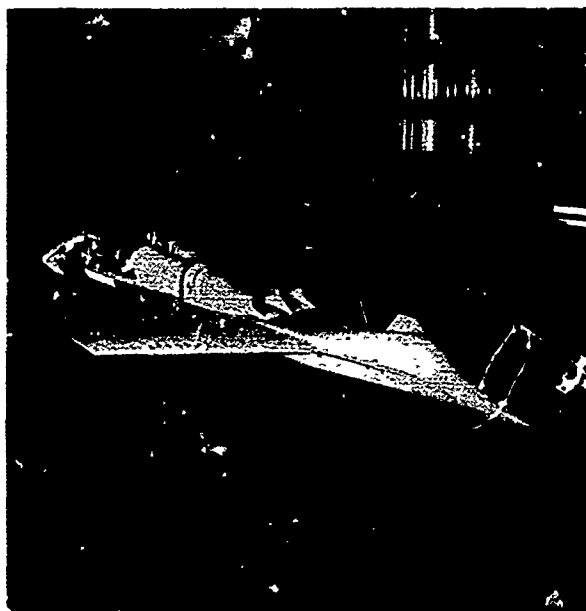
Figure 35. Above the wing inlet study in the Ames 11-ft tunnel (Ref. 42).
