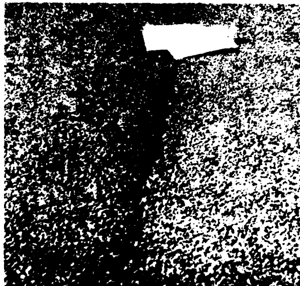
Figure 7c. High-severity crack in PFS pavement: Average raveled area around the crack is greater than 1 in. wide.
