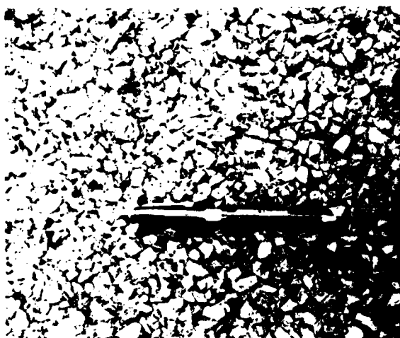
Figure 8a. Example 1 of a typical PFS surface with no raveling and weathering.
