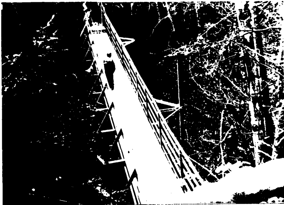
PHOTO #2: Top of dam from left abutment
