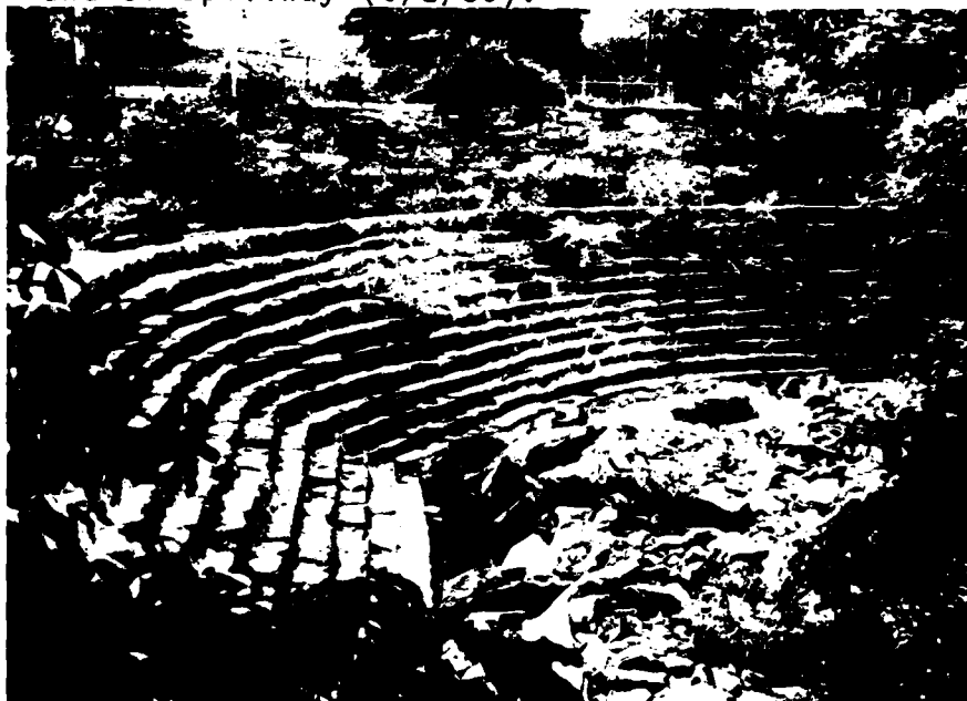
Photo 4 - View of spillway from right end. Note riprap displacement at toe and vegetation growth on downstream face (6/2/80).
