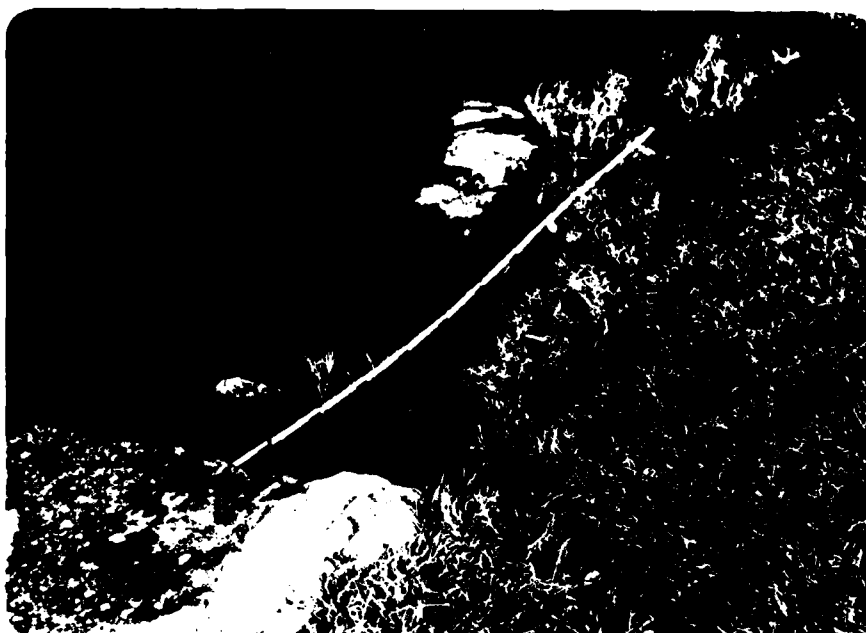
10 Sta 3+90, upstream face has been displaced, rule extended 6 feet.
