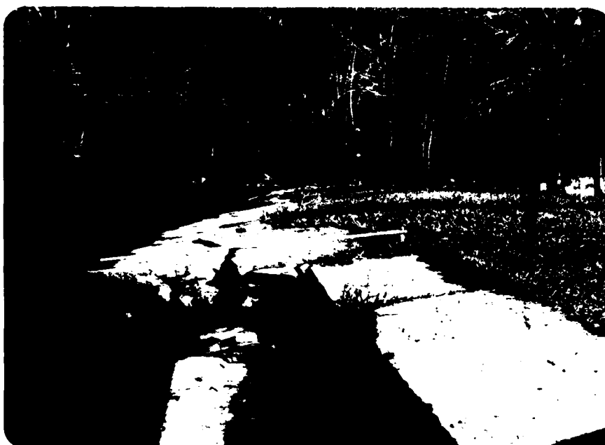
9 Sta 3+00, looking along upstream edge of crest, displacement toward reservoir, up to 4 inches vertical displacement between top of wall and adjacent soil crest.
