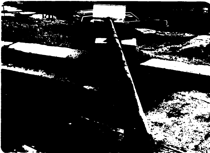
6 Sta 2+73, looking along upstream face of wall; displacement of concrete slabs beneath pipe 5 inches downward.
