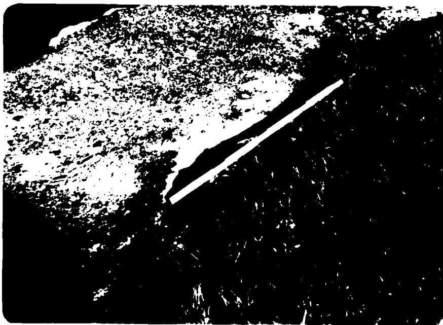
4 Sta 1+00, crack in concrete along upstream edge, 1 foot long, 3 inches wide, 1 foot deep, 3 feet from edge of upstream wall.
