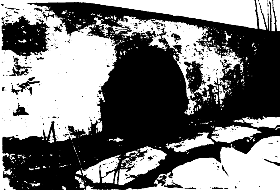
PHOTO C-12 Left outlet works conduit and stone masonry foundation ruins at downstream toe of dam.
