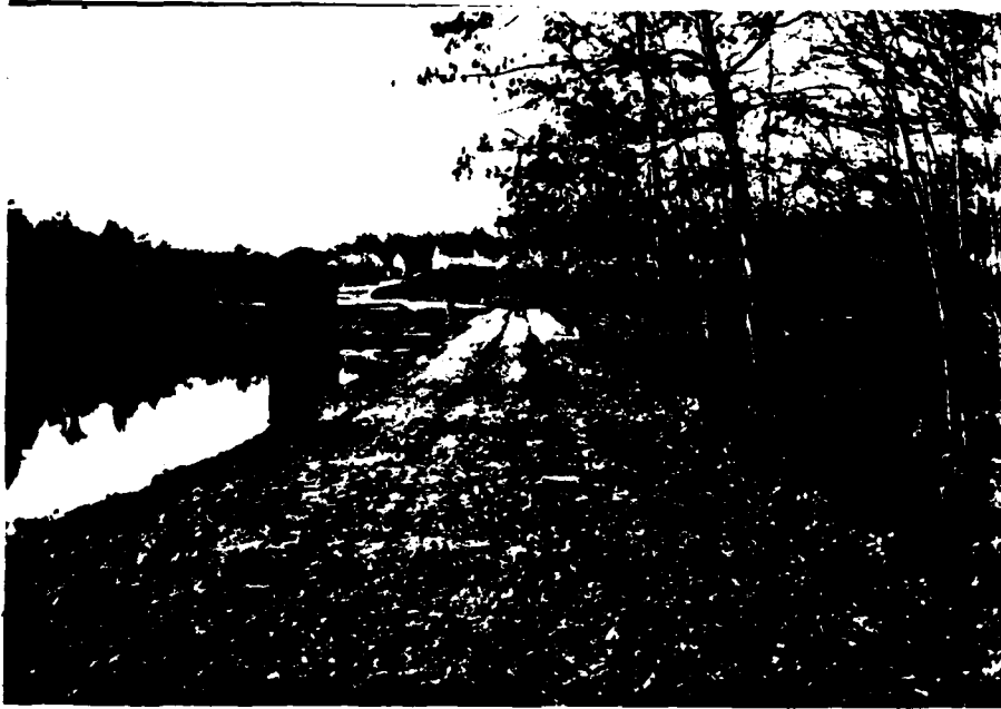
C-3 CREST OF MAIN EMBANKMENT.
