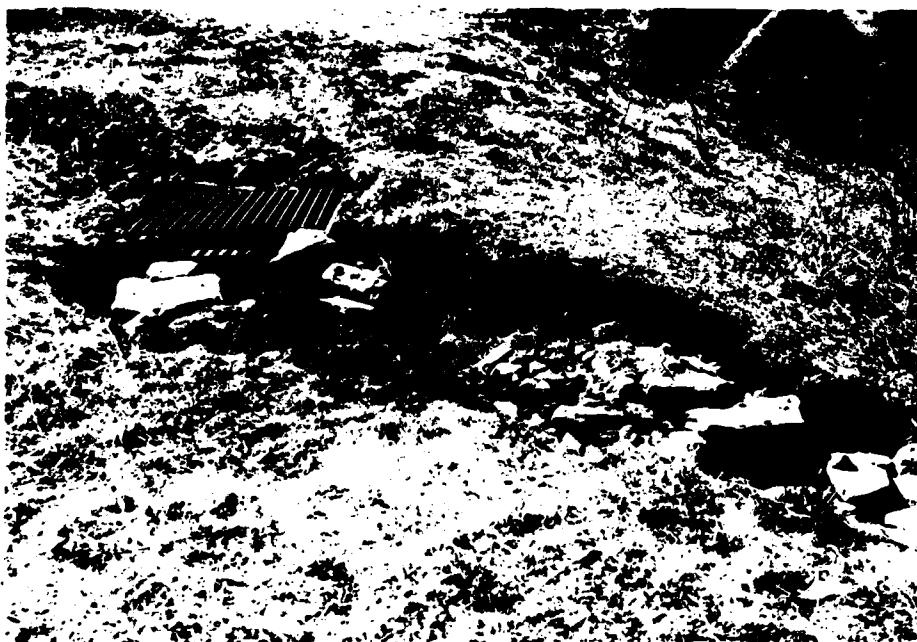
C-12 SURFACE EROSION FROM IMPROPER DRAINAGE FACILITY ADJACENT TO SPILLWAY
