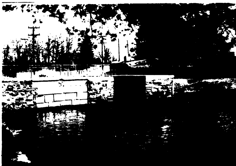
C-7 UPSTREAM FACE OF DAM AT LEFT ABUTMENT; BLOCKED PENSTOCK OPENING AT LEFT - APPROACH TO CONTROL GATES - MIDDLE - SPILLWAY AT RIGHT
