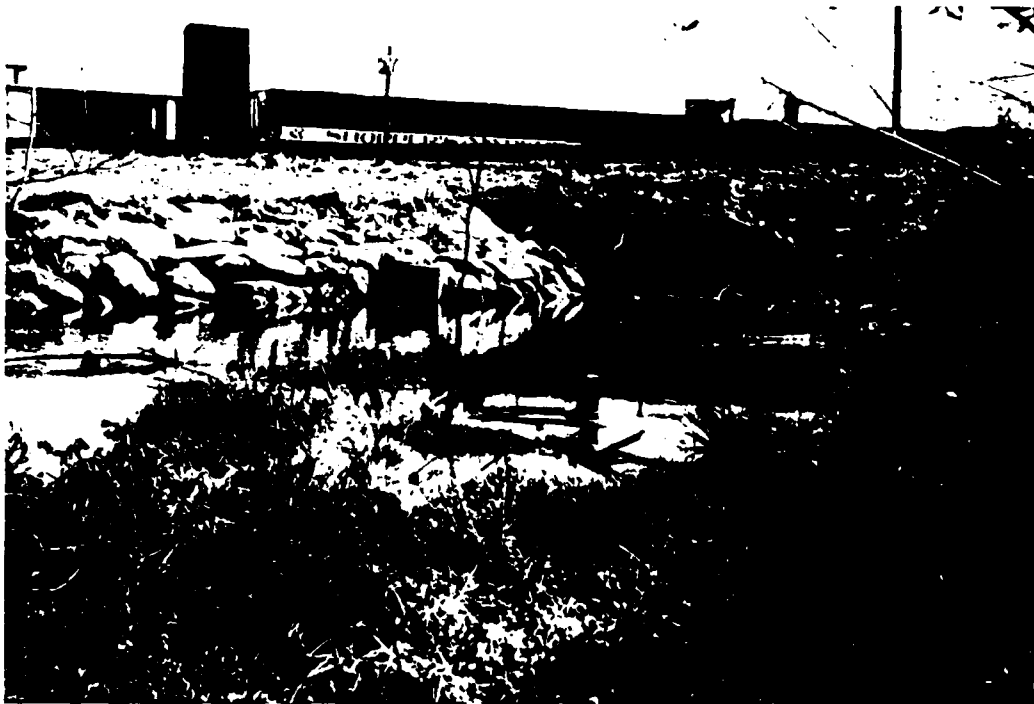
9a. AT INLET. NOTE RIPRAP SLOPE.
