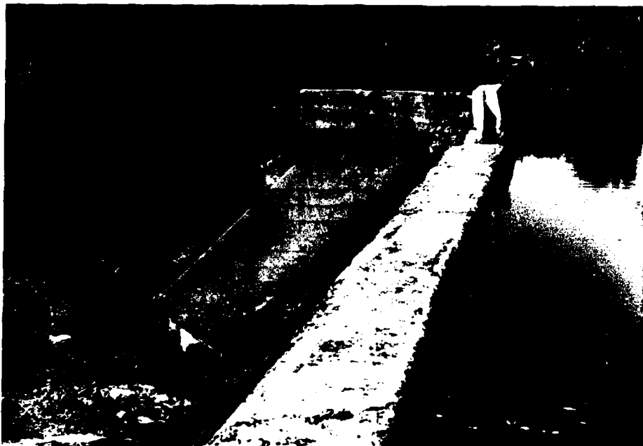
8. RIGHT SIDEWALL OF CANAL SPILLWAY.
