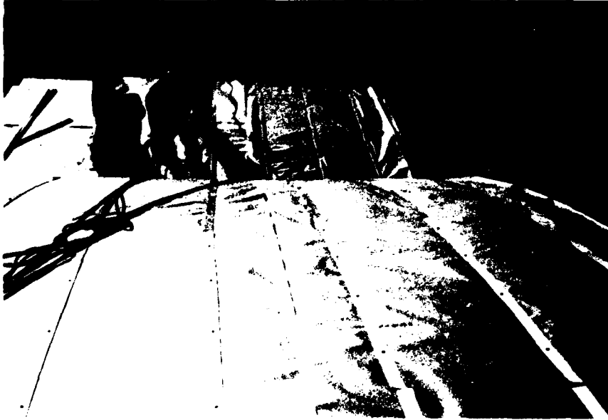
Figure 28. Batten strips installed above slip sheet.
